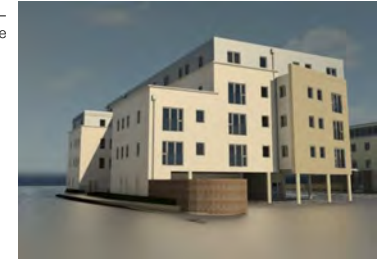
Approved View – South West / Brougham Hayes Façade
