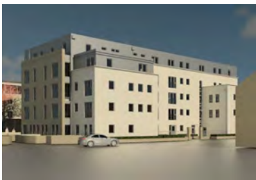
Approved View – North West / Brougham Hayes Façade
