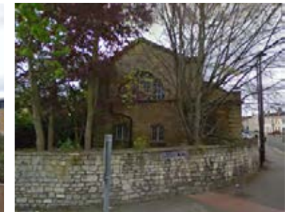
Images of the existing building
